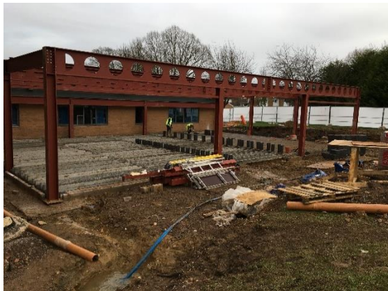
Foundations and steelwork completed
