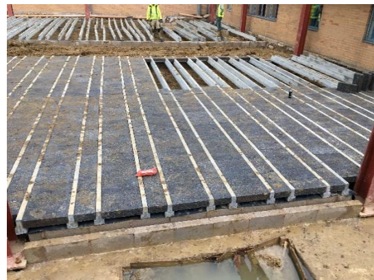
Floor construction in progress
